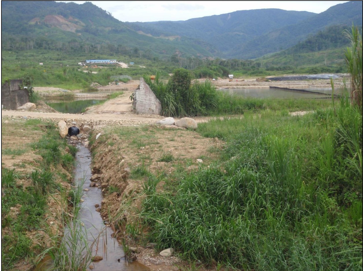
Figure 19c. The grey colour of the discharge from the sedimentation ponds shows that the sedimentation ponds are not functioning (Quishpe Lozano et al., 2018). Photo taken by the author on 6 November 2018.
