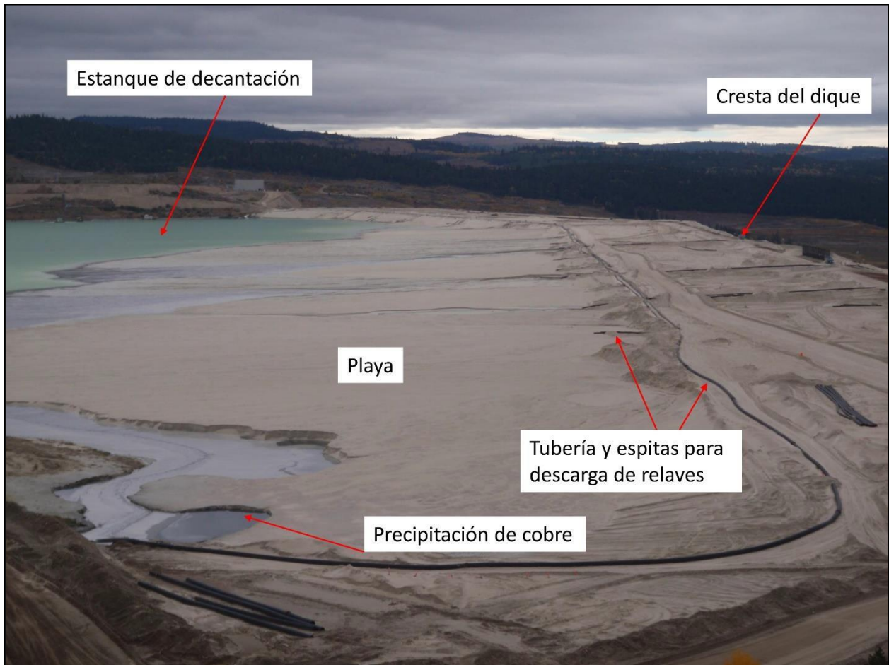
Figure 4. At the Highland Valley copper mine tailings storage facility in British Columbia, wet tailings are discharged in the upstream direction from a pipe and spigots along the dam crest. Larger particles (sands) are deposited near the dam to form a beach. Smaller particles (silts) are transported further away from the dam to form a settling pond. Copper precipitation in the tailings pond indicates incomplete extraction of copper from the ore. The narrow beach (especially on the opposite side, where the beach is almost non-existent) makes the dam susceptible to flood failure. Photo taken by the author on 27 September 2018.
