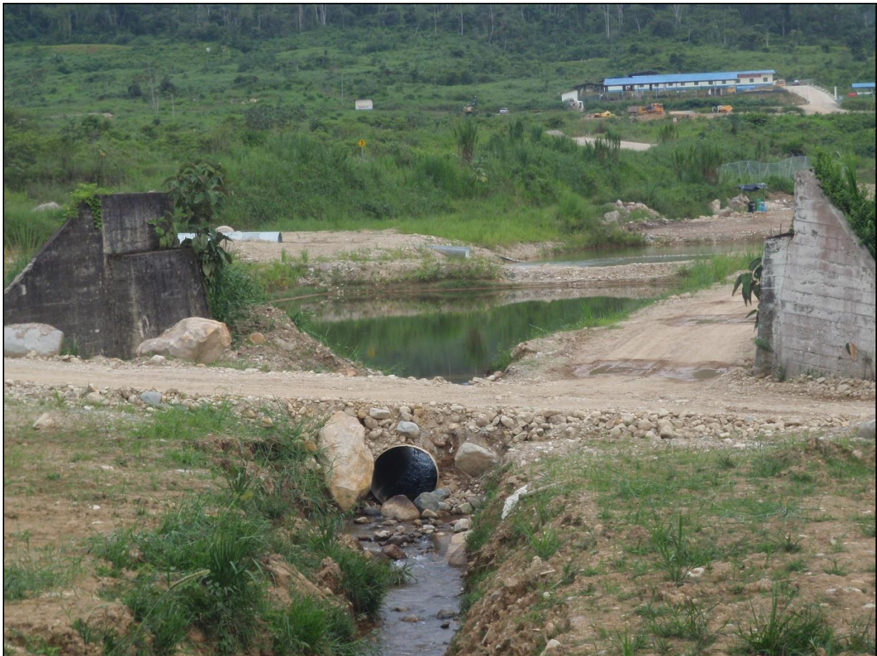
Figure 19a. Overflow from the sedimentation ponds for the Tundayme tailings dam is discharged into a pipe and flows into the Quimi River (see Figure 11). Photo taken by the author on 6 November 2018.
