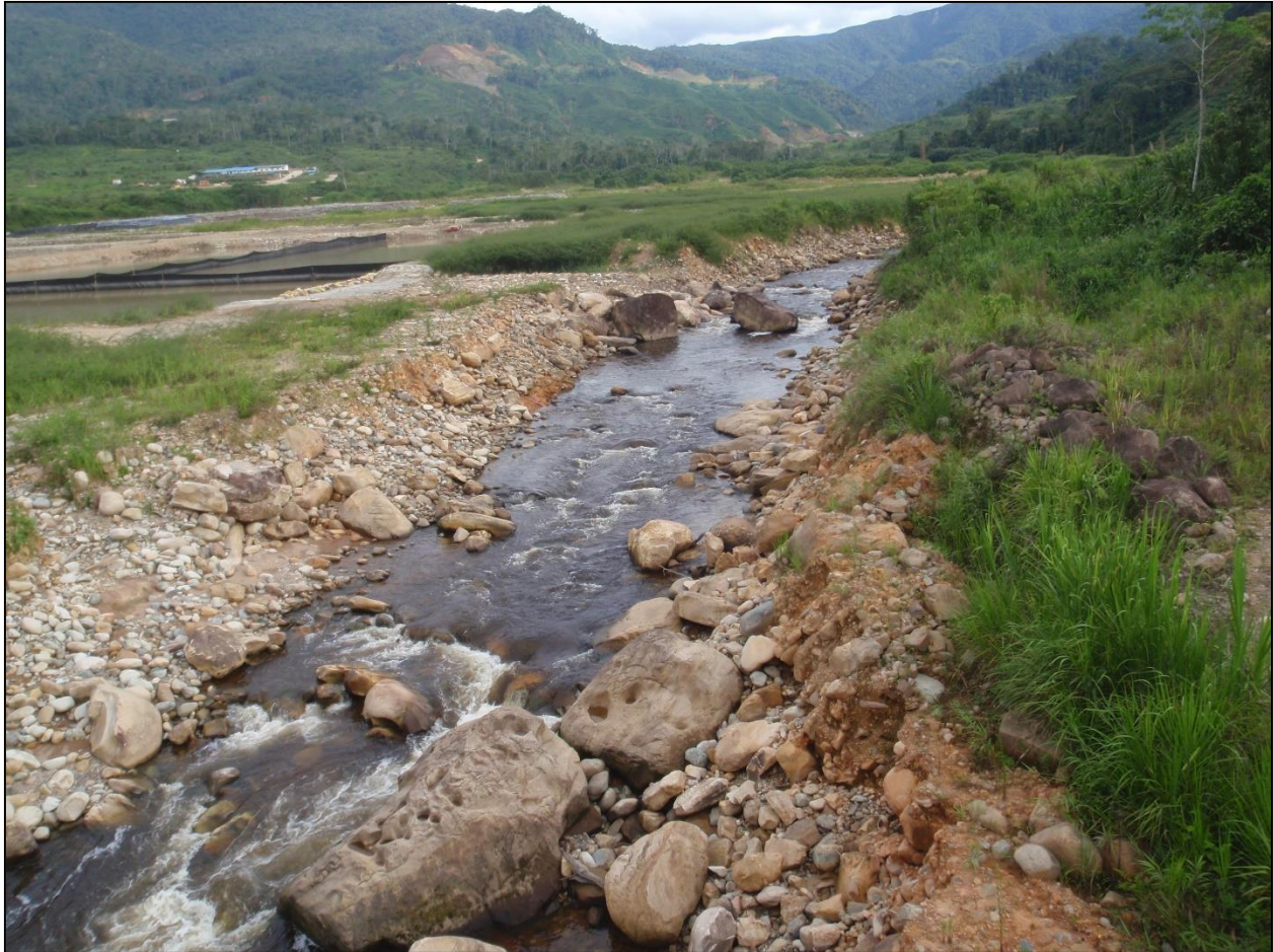
Figure 20. According to a complaint by the provincial government of Zamora Chinchipe (Quishpe Lozano et al., 2018), "Here the extraction of stone material was taking place in a portion of the Tundayme River [shown above]. As in the Quimi and Waywayme rivers [see Figures 2 and 11], the extraction of stone material in this area is not carried out within any mining concession for the exploitation of aggregates and stone...It is worth noting that in the review of the national Mining Cadastre, no mining titles for the exploitation of stone material within the Mirador project in the aforementioned area are registered". A possible explanation for the illegal extraction of construction material from the rivers is the lack of other sources of construction material. A shortage of construction material could also explain the change from centreline construction to upstream construction (see Figure 16) and the excessively steep embankment of the initial embankment (see Figure 17). Photo taken by the author on 6 November 2018.
