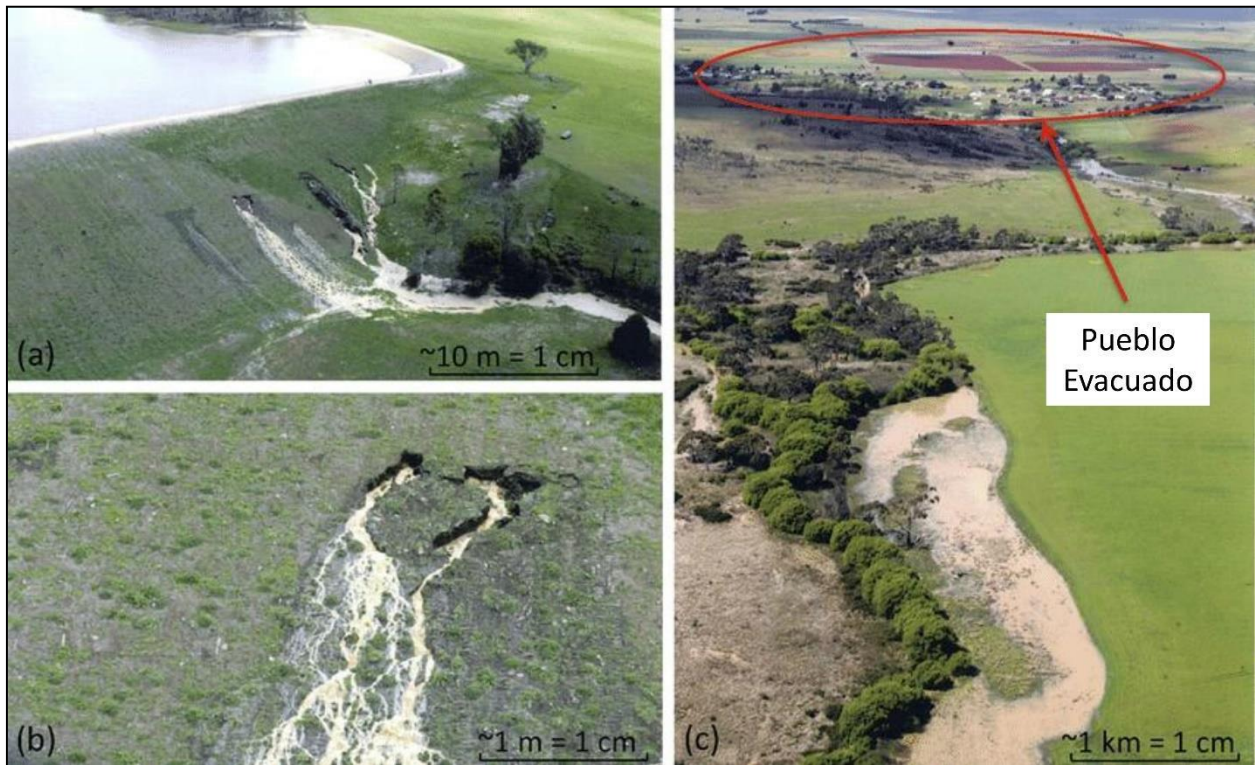
Figure 7. Internal erosion (also called channelisation) caused the failure of an earth dam in Tunbridge, Australia, in 2005. During internal erosion, seepage transports solid particles out of the dam so that the dam loses structural integrity. Internal erosion can be considered a type of liquefaction because the water carries the load of the dam. Internal erosion is promoted by an excessively steep embankment slope and the resulting high hydraulic gradient, which forces water to flow through the dam. Photo modified from Fisher et al. (2017).
