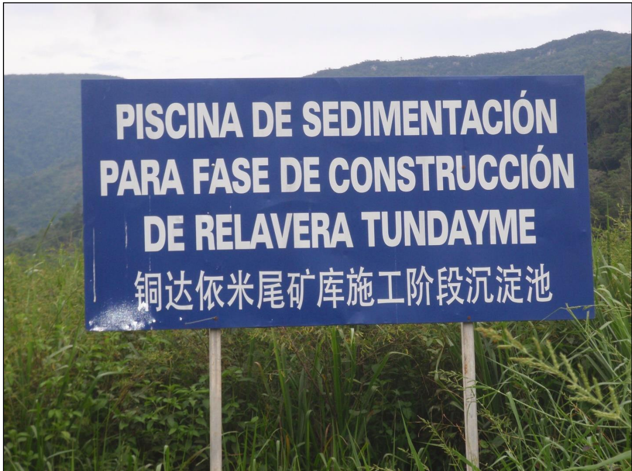
Figure 18. The sign makes it clear that both the Quimi tailings dam (see Figures 1, 16 and 17) and the Tundayme tailings dam are currently under construction. This is inconsistent with the Environmental Impact Assessment (Cardno, 2014a), which listed the two tailings ponds as alternatives. Photo taken by the author on 6 November 2018.
