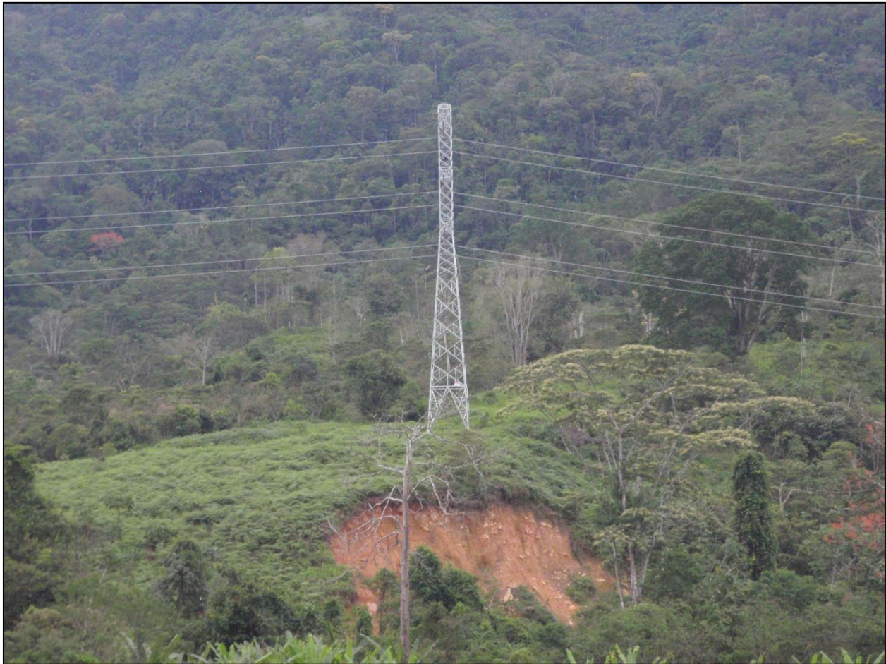
Figure 15. The high erosion rate in the project area is indicated by the landslide scar below a transmission tower on the north bank of the Quimi River (see Figure 11), opposite the Quimi tailings dam. Photo taken by the author on 6 November 2018.
