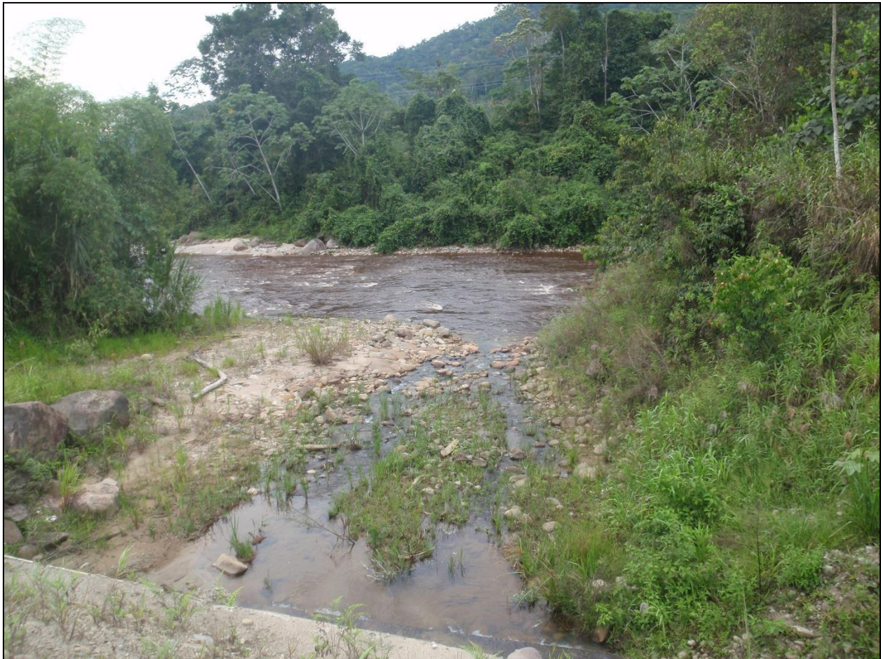
Figure 19b. The pipeline from the sedimentation ponds discharges directly into the Quimi River. Photo taken by the author on 6 November 2018.
